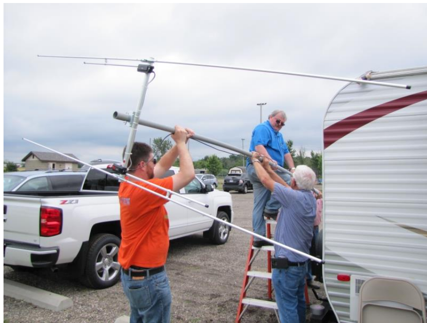
Folks working on the 6 meter beam
